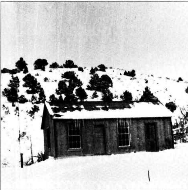
14: Schoolhouse at the Baumanns' McCluskey Creek ranch, Eureka County, Nevada, 1923-24 school year. Pietrina Damele Etchegaray, the teacher, had her living quarters on one side of the building and the school was on the other side.
