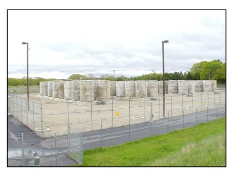
Figure 14. Dry Cask Storage Facility at the Decommissioned Maine Yankee Reactor Site (*source*: <u>http://www.maineyankee.com</u>)
