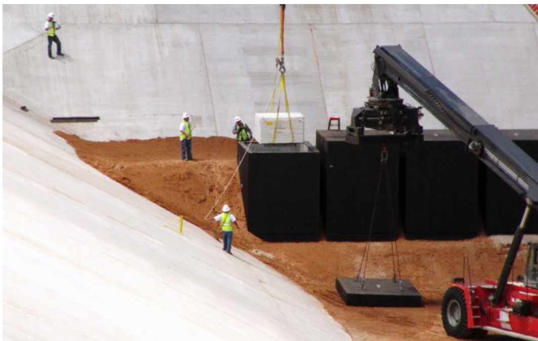
In this June 6, 2013 file photo, crews from Waste Control Specialists load the first of two containers with low-level radioactive waste from Los Alamos National Laboratory in New Mexico, into a reinforced 8-inch-thick concrete container at the 90-acre federal dump where it will remain forever, near Andrews, Texas.
